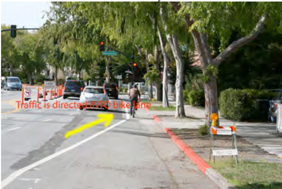
Looking North on Middlefield at Mayview Signal: Traffic is directed into the bike lane at the pinch point - VTA busses commonly veer into the bike lane now. Note the vehicle's reaction to the bicyclist.
